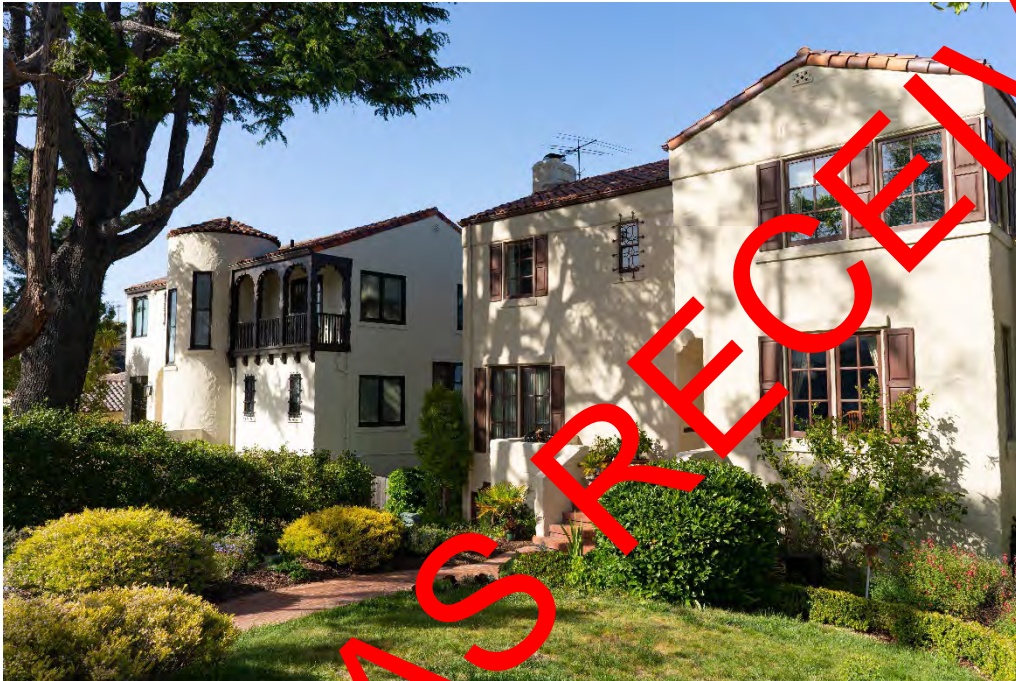
11 of 31. 321 and 327 Georgetown Avenue. Camera facing north.
