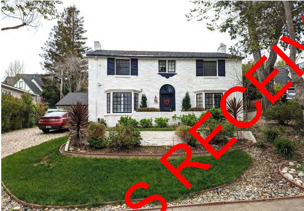
19 of 31. 511 Parrott Drive. Camera facing southeast.
