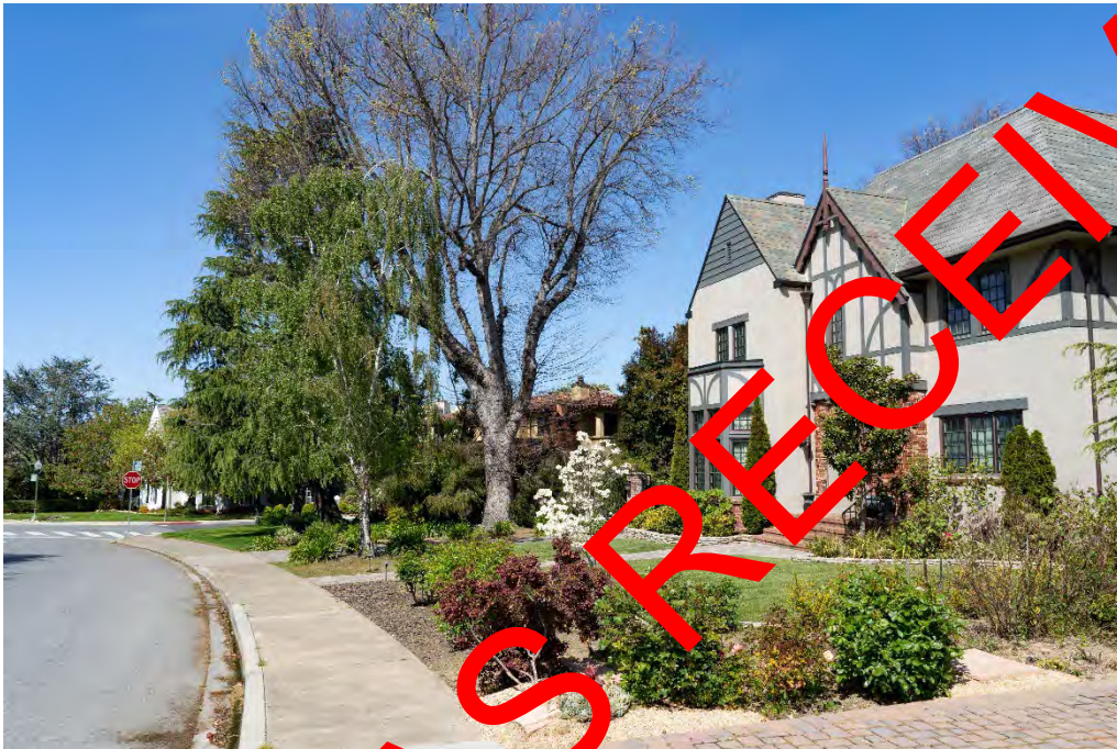
5 of 31. 311 Barnett Drive. Camera facing northeast.
